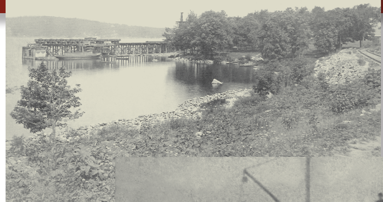
Ore Docks at Nolan's Point
